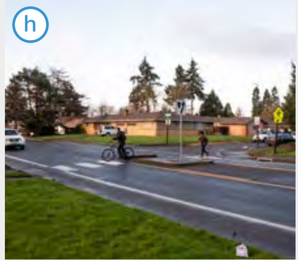
Refuge islands protect pedestrians and cyclists as they cross Echo Hollow Rd at Murnane St.
