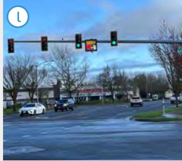
For bicyclists traveling north on Echo Hollow Rd and turning west onto Barger Dr, there is a newly-constructed staged left turn that routes them onto the separated cycle track on the north side of Barger Dr. However, the signage explaining this maneuver is located too close to the intersection for bicyclists to take note of and follow the instructions.
