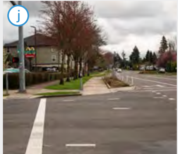
The bicycle facilities on Barger Dr are buffered from motorists at the intersection by a landscaped barrier. The City of Eugene recently replaced a right turn lane with these new curbs, plastic bollards, and a rain swale.
