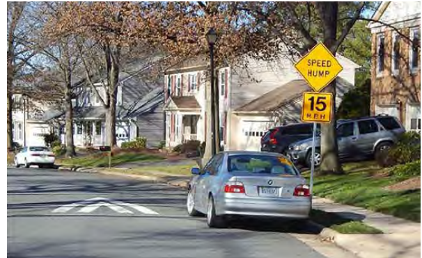
Speed humps help to slow traffic.
