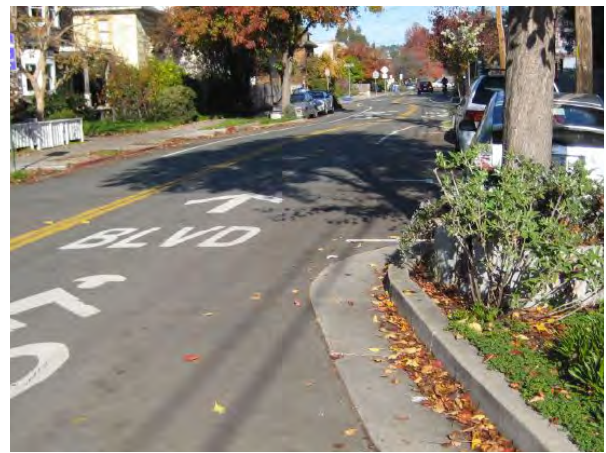
Curb extensions narrow the roadway, and pavement markings reinforce the greenway designation.
