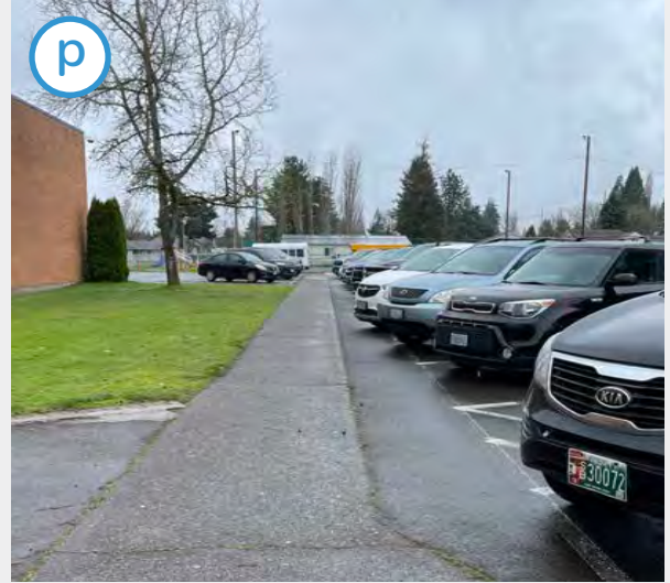
Most stalls in the high school parking lot lack concrete curbs to prevent encroaching into the pedestrian space.
