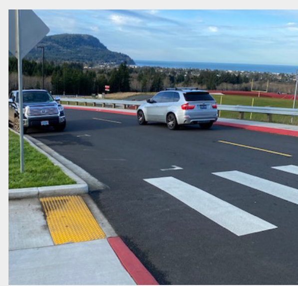
Crosswalk at the top of the hill on Spruce Dr. Vehicles are allowed to park along this row, however the parking spaces closest to the crosswalk block oncoming vehicles from seeing pedestrians crossing the street.
