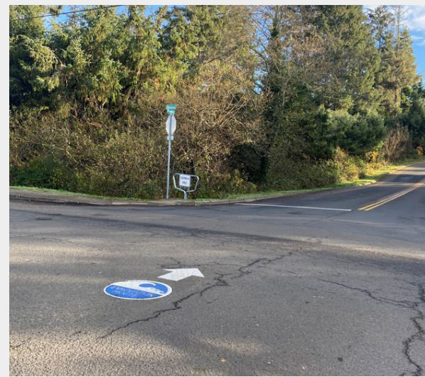
At the intersection of Wahanna Rd and Broadway St, there are no marked crossings. Current stop lines are faded and not highly visible. There are also no sidewalks on the west side of Wahanna Rd.
