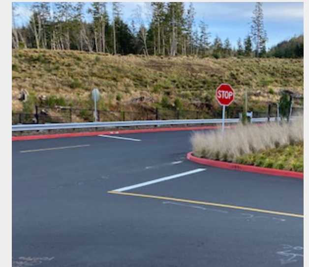
Intersection at the front of the middle/high school, where the front parking lot meets Spruce Dr. There is no crosswalk at this stop sign, causing students to cross the street at different locations.
