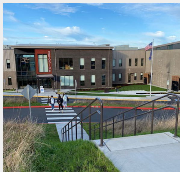
Crosswalks from the parking lot to the rear entrance of campus. The majority of students park in this parking lot.
