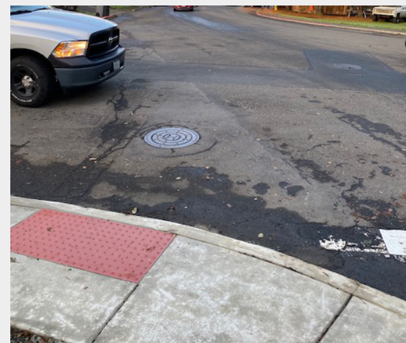
Vehicles travel down Alder Dr, turning right onto Spruce Dr to access both schools. Many parents drop-off/pick-up in nearby neighborhoods and use this route. There is a need for lighting in this area as well as improved crosswalks, curb ramps, sidewalk alignment, and improved stop lines.
