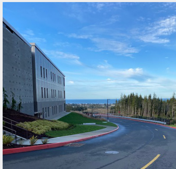
Students trying to access the rear entrance of the middle/high school must travel around the side of the building and up stairs. This is the only way to access this entrance, however students often travel the shortest distance and walk directly in the road.
