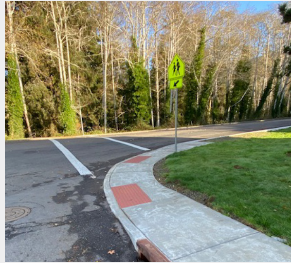
Curb ramps at the intersection of Spruce Dr and Alder Dr to not align with crossing. Crosswalks are also not high-visibility, making it more difficult for vehicles to see students crossing.
