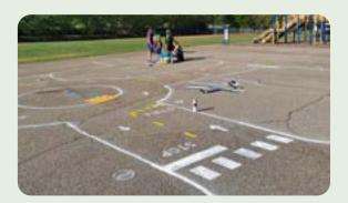
Street network and traffic features are created from materials that wear away such as spray marking paint. Typically, an installation remains in place for several weeks to months.
